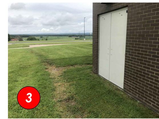
INSTALL CODE REQUIRED CONCRETE PADS AT EGRESS DOORS
