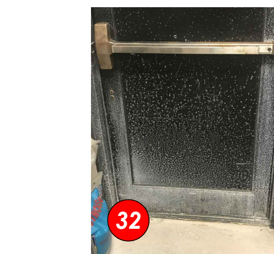
REPLACE EXTERIOR DOOR AT THE POOL CHEMICAL STORAGE ROOM
