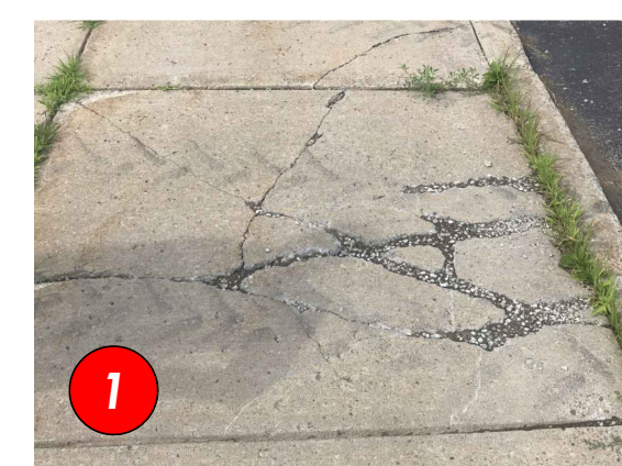
REPLACE DETERIORATED SECTIONS OF EXISTING CONCRETE SIDEWALKS
