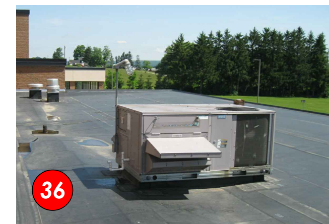
REPLACE EXISTING ROOFTOP AIR HANDLING UNITS AND EXHAUST FANS
